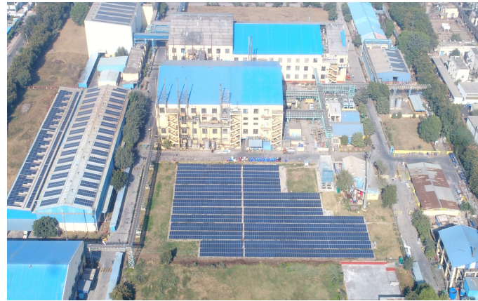
Solar Panel installation at Bawal Plant
